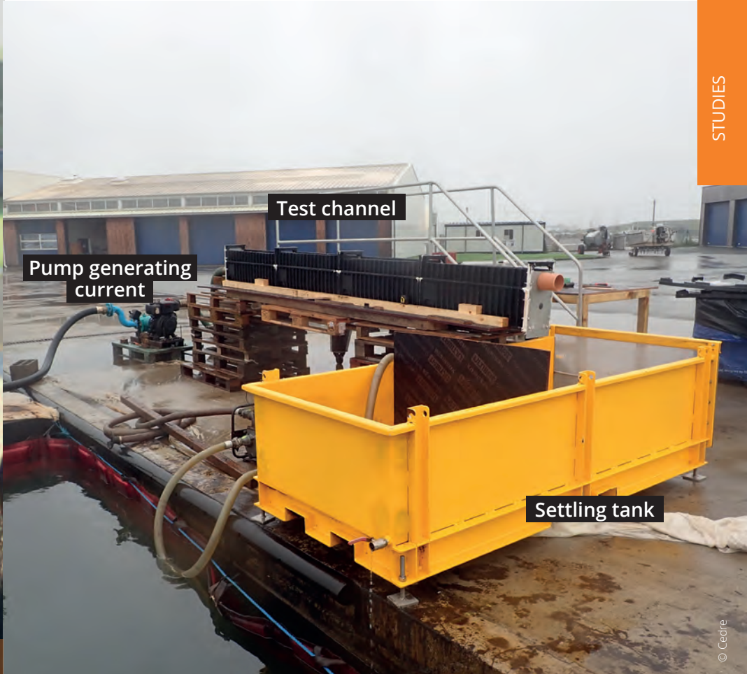
▲ Installing the filtration testing system
