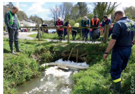
△ Designing and building custom-made booms in the natural environment on the banks of the Penfeld river
