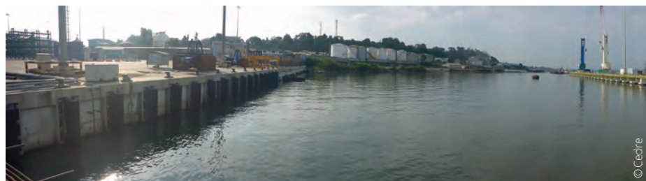
^ SGEPP oil storage facility in Owendo, Libreville - Gabon
