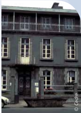
Our first offices at the port of Brest
