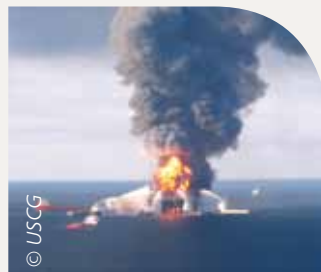
Deepwater Horizon rig on fire
