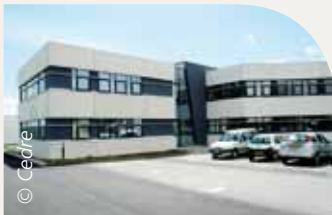
The new emergency response centre
