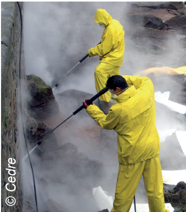
Booms and sheets deployed to trap thermal washing effluents
