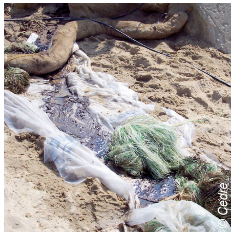
Booms and mops (trapping of cleanup effluents)
