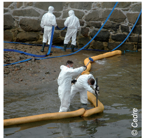
Deployment of sorbent booms before cleanup starts
