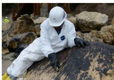
Left: Evacuating lightly oiled sand in sacks (Refugio State Beach, 23rd May); Above: scraping splashes off rocks (Source: USCG)
