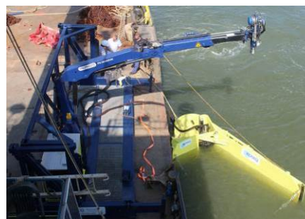
Deploying the Koseq Compact 502 (Source: Koseq)
