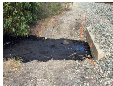
Left: Close-up of the breach in the line (Source: PHMSA); Right: Visible crude oil leak at a drainage culvert (University of California Santa Barbara)
