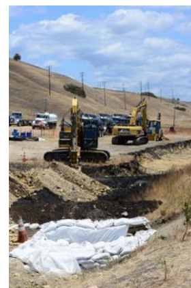
22/05/2015: Excavating soil near to the spill point (Source: USCG)
