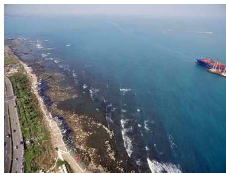
Late March: Aerial view of the wreck of the TS Taipei and the nearby exposed shoreline where clean-up operations were being conducted (Source: Taiwan Environmental Protection Agency)
