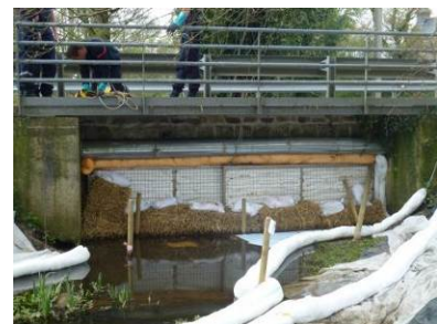
Filter system (straw and sorbents in a wire structure) 1.5 km downstream of the leak (Source: Cedre)
