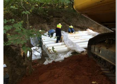
Left: Areas of high concentrations of petrol in the contaminated pond: Right: Construction of bunds with underflow pipes at a natural weir in the pond (Source: US EPA)
