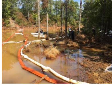
Left: Petrol containment/recovery sites along the banks; Right: Liquid waste storage in Frac Tanks, to the rear of the clean-up sites (Source: US EPA)
