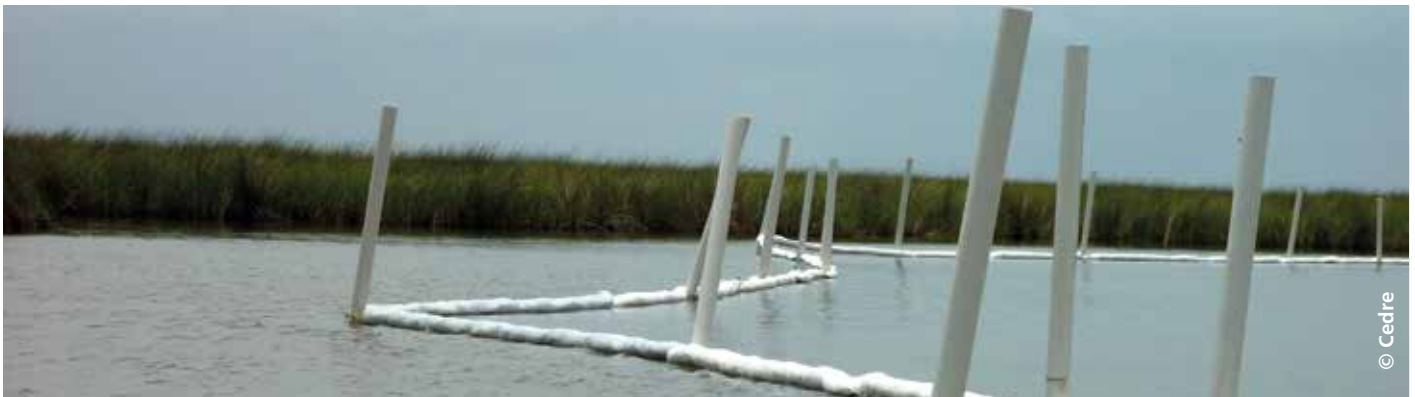
☾ Sorbent booms laid to protect the shoreline during the Deepwater Horizon spill
