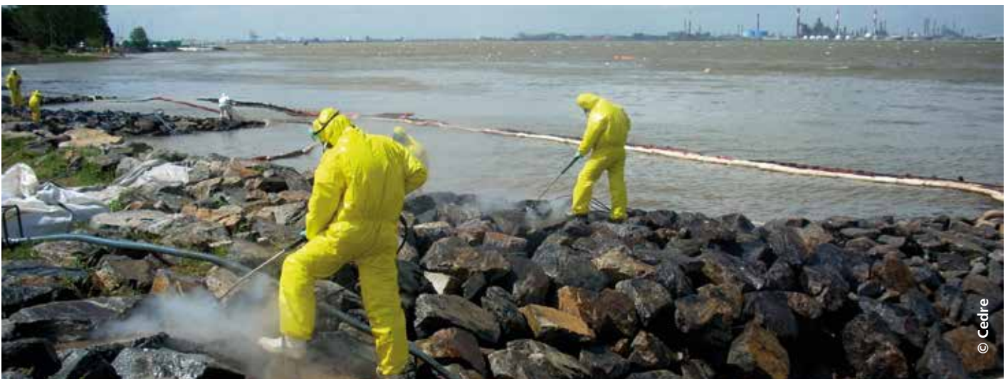
Pressure washing riprap
