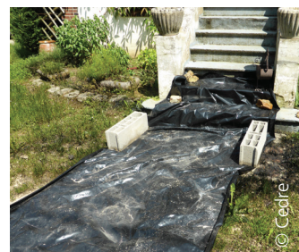
Cleaning up contaminated gardens
